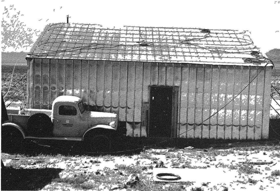
Fig 1 1 — General view of Butler building
